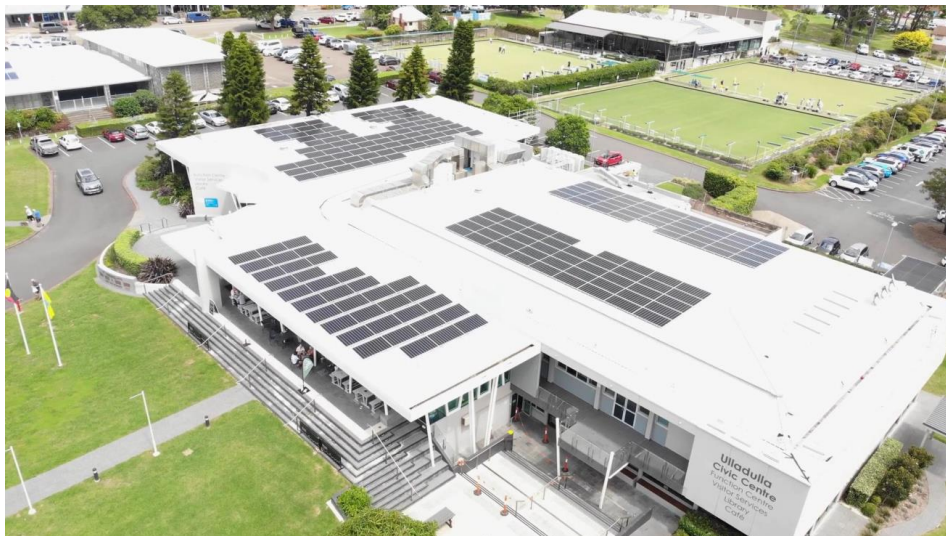
A 100-kW solar PV system installed on the Ulladulla Civic Centre roof in 2023
