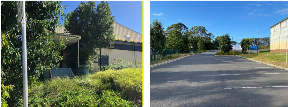
Figure 13. Photographs of existing entry to Basketball Stadium & affected vegetation along the eastern side of existing building
