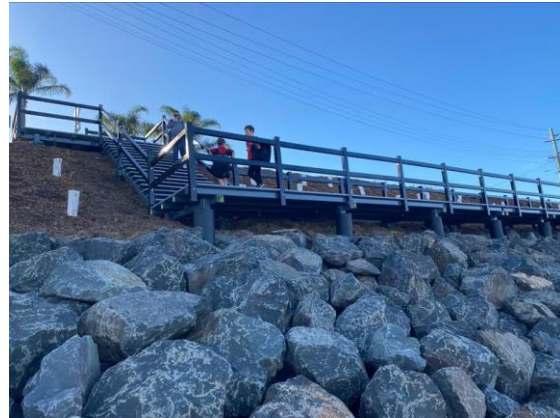
Rock revetment and segment of the boardwalk
