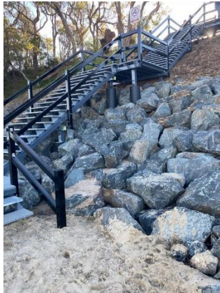
Access stairs and rock revetment
