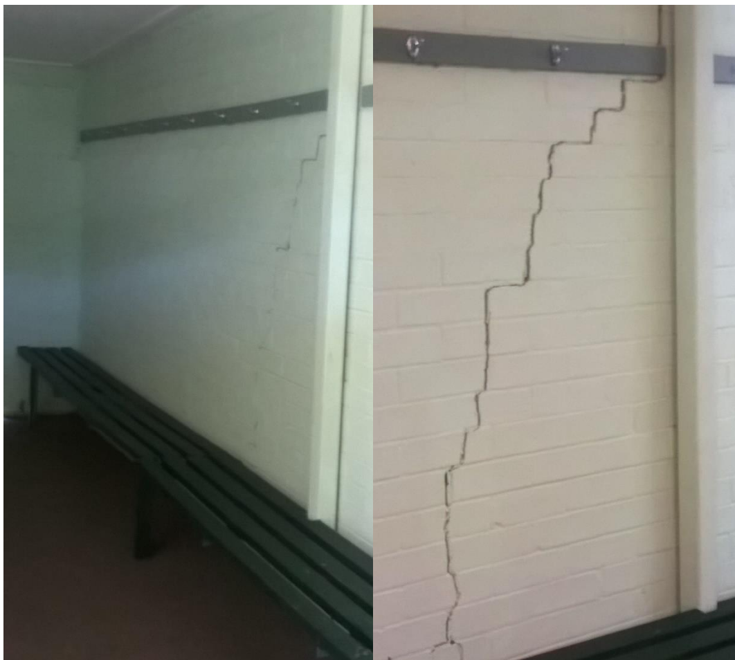
Change room and cracked walls
