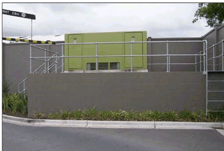
Figure 51 - Example substation raised above 1:100 flood level
