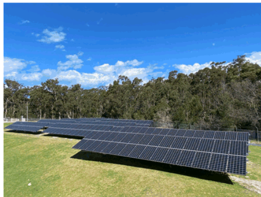
Vincentia WWTP 95 kW ground-mounted solar PV array
