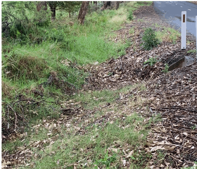
Photo 5: Photo taken on Beach Road of the culvert mentioned in PP technical report 'Appendix F – Water Cycle Management Plan' which is UPHILL from gully and 'Dam 1' overflow. In fact water would likely flow in the opposite direction to that stated in the PP.
