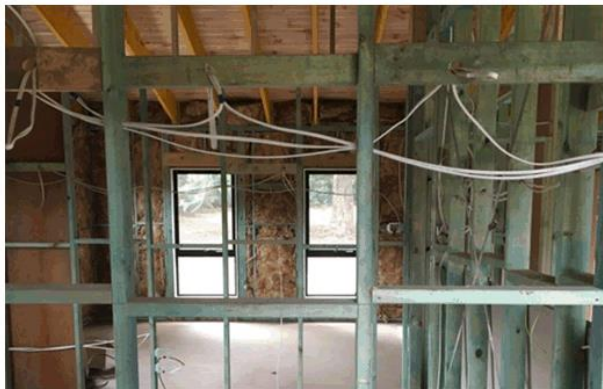
Electric Wiring
