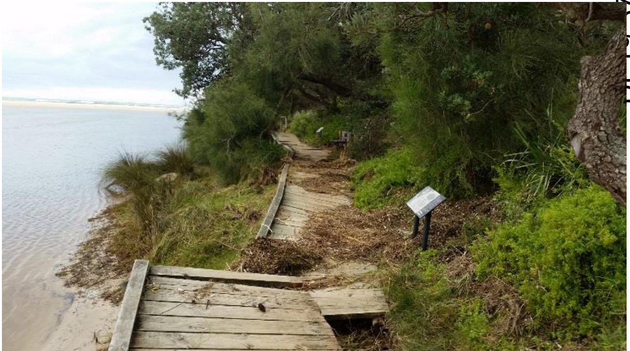
Figure 1: Lake Tabourie Boardwalk, damaged following East Coast Low, July 2016
