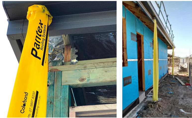
Figure 9 - Typical detailing for temporary downpipes
