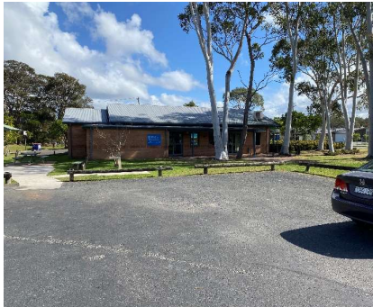
Eastern side of Callala Bay Community Hall & adjacent carparking
