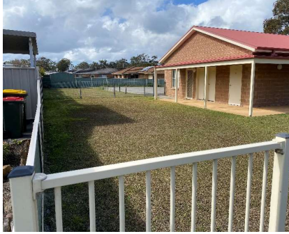
Northern façade of Anglican Church
