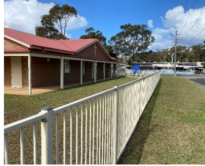
Western façade of Anglican Church (school to south of Emmett St)
