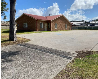
Eastern façade of Anglican Church (carpark)
