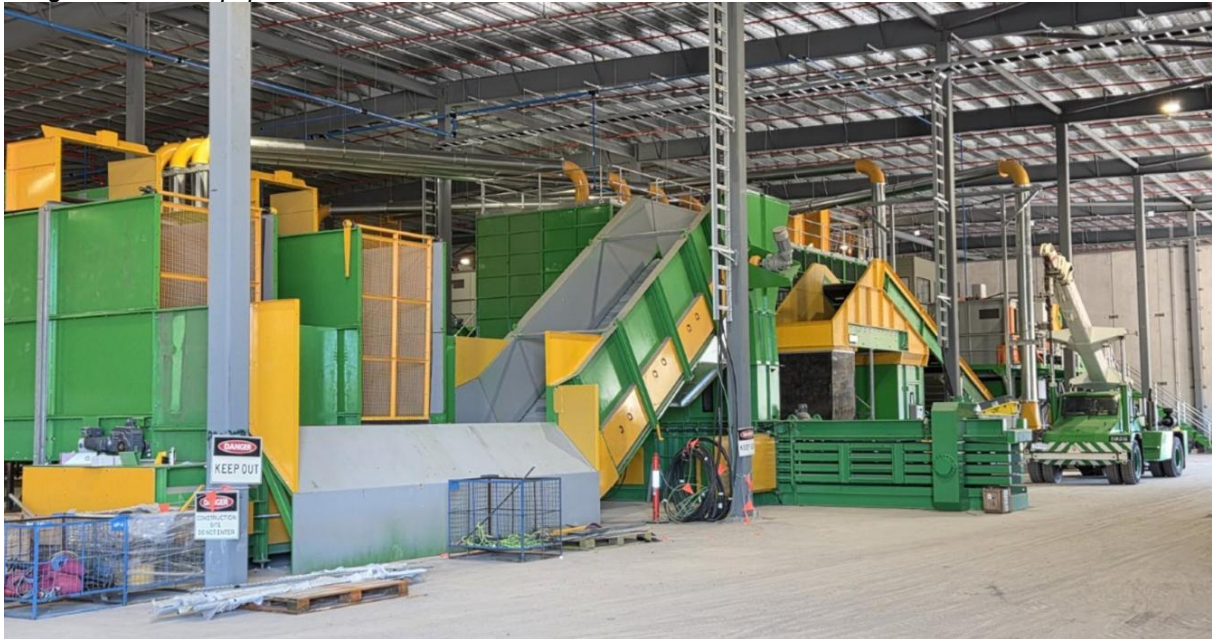
Image 1 – MRF Equipment Installation
