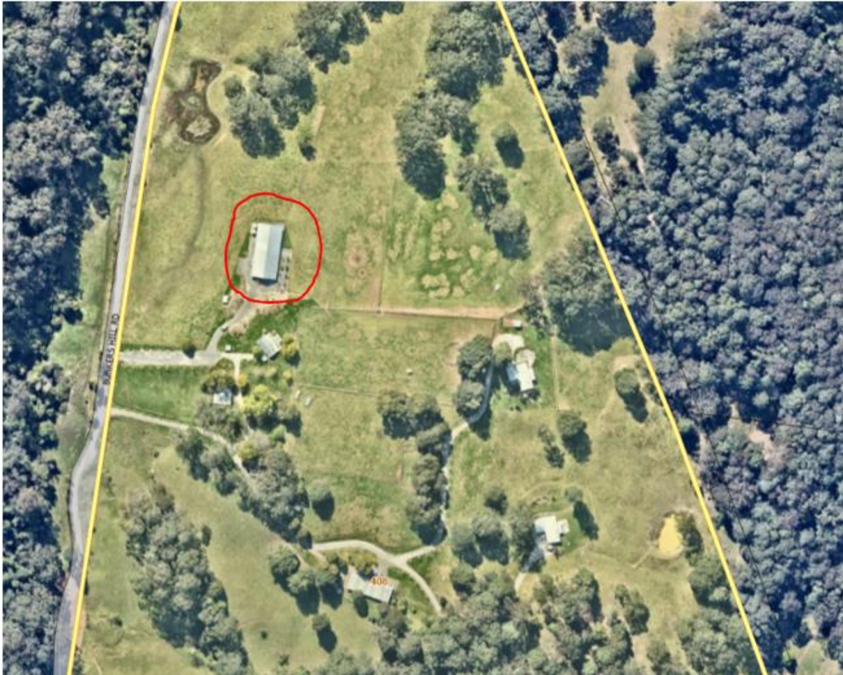
Figure 2: Aerial imagery of development site. Building proposed to be used as dwelling house circled in red.
