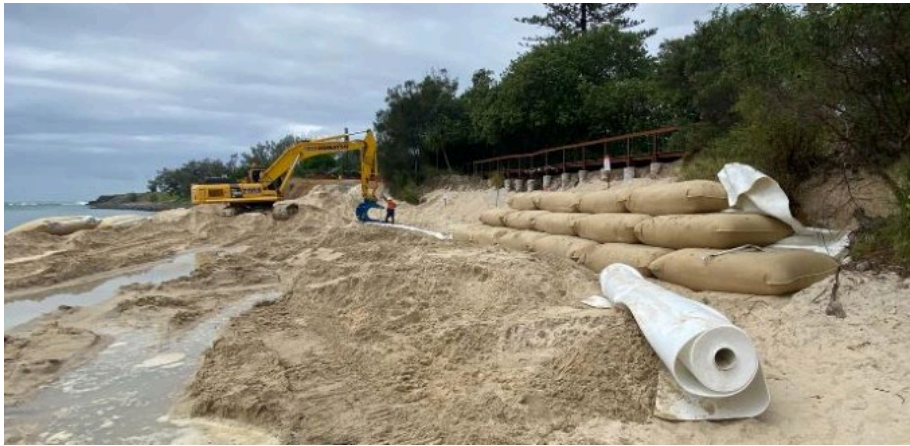
Figure C-6 Example of Interim 'Soft Works' in the Form of Temporary Geotextile Sand Containers. Photo Sourced from Mulcahey et al (2023)
