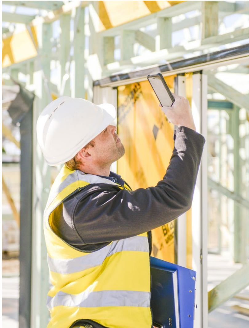
Construction site inspections
