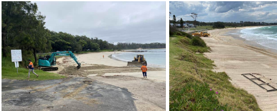
Figure C-1 Emergency beach scraping works undertaken by Council after storm events. Left: Bandalong Boat Harbour, April 2022. Right: Mollymook Beach, June 2020. Image source: SCC
