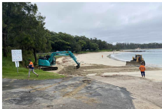
Figure 2-8 Emergency beach scraping works undertaken by Council after storm events. Left: Bendalong Boat Harbour, April 2022. Right: Mollymook Beach, June 2020. Image source: SCC
