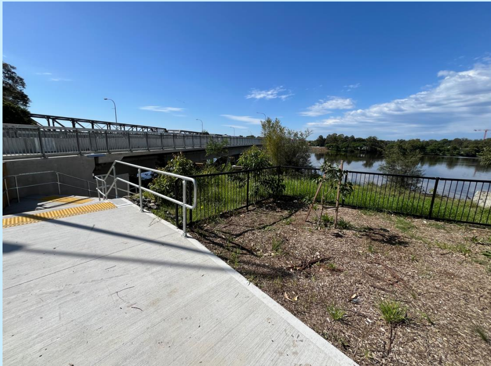
Northern side of the River – Illaroo Road (south side)
