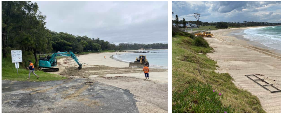
Figure 2-8 Emergency beach scraping works undertaken by Council after storm events. Left: Bandalong Boat Harbour, April 2022. Right: Mollymook Beach, June 2020. Image source: SCC
