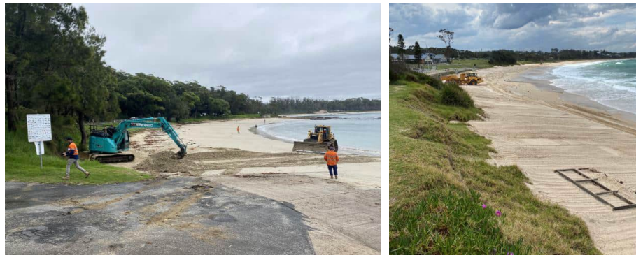
Figure C-1 Emergency beach scraping works undertaken by Council after storm events. Left: Bendalong Boat Harbour, April 2022. Right: Mollymook Beach, June 2020. Image source: SCC
