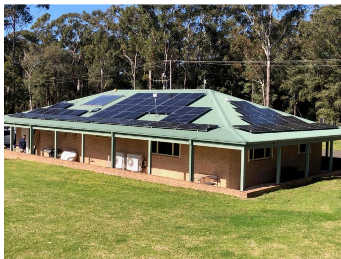
A 20-kW solar PV installation at St Georges Basin Wastewater Treatment Plant
