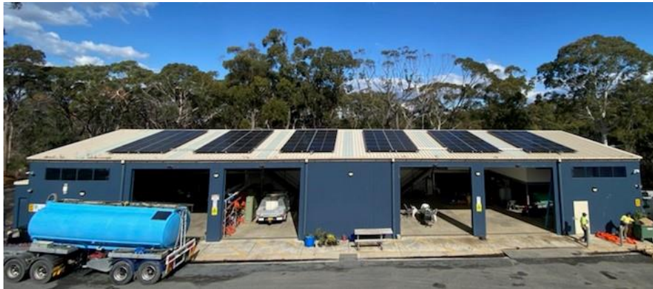
A 30-kW solar PV system installed on the Shoalwater Shed roof at the Ulladulla Works Depot in 2022
