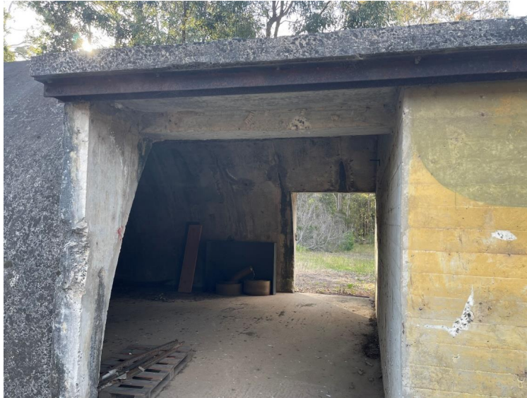
Figure 35. Detail of the entrance to Torpedo Storage Bunker A3. Steel doors would have run along the steel rail.
