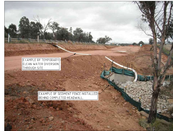
PHOTO 1: TEMPORARY CLEAN WATER DIVERSION AND SEDIMENT FENCE BEHIND COMPLETED HEADWALL
