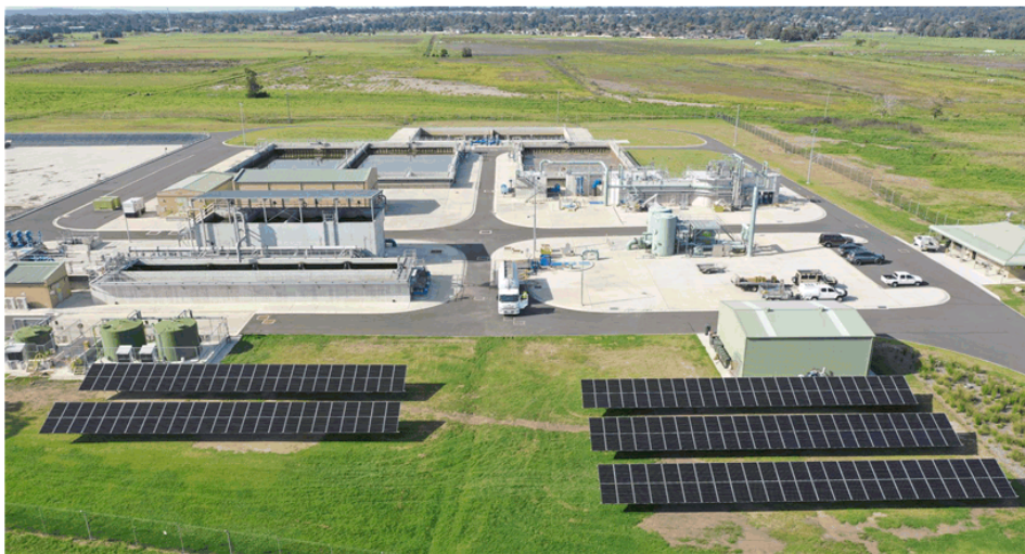
Photo - A new 100 kW ground-mounted solar PV system installed at Nowra Wastewater Treatment Plant
