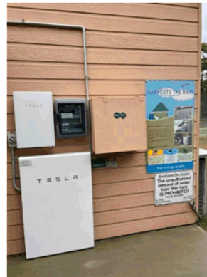
Solar PV and Battery installations at Berry and Kioloa as part of Council's Recovery into Resilience project supplying secondary backup power during grid outages
