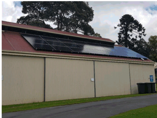
Solar PV and Battery installations at Berry and Kioloa as part of Council's Recovery into Resilience project supplying secondary backup power during grid outages
