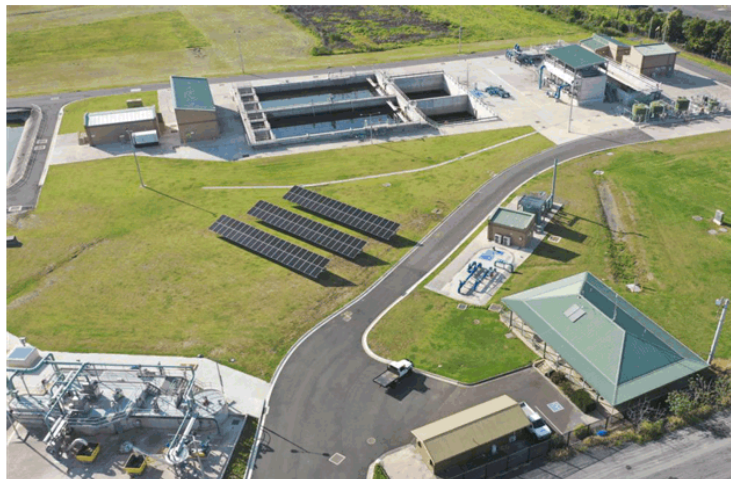
A new 50 kW solar PV system installed at Bomaderry Wastewater Treatment Plant
