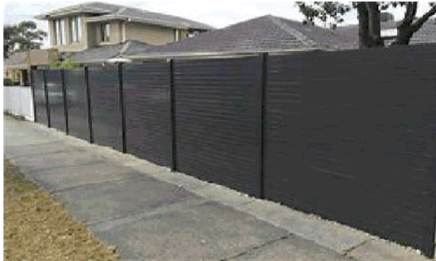
Fence Type 3 – Aluminium Slat Fence 1.2m high
