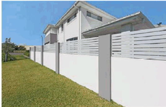
Fence Type 2 – Modular Wall – Estate Wall 2.2m High proposed along the highway frontage with return in Pitman Ave east of the proposed BBQ area.
