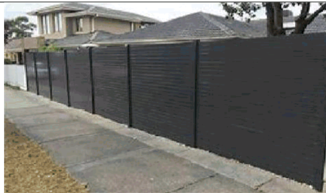
Fence Type 3 – Aluminium Slat Fence 1.2m high
