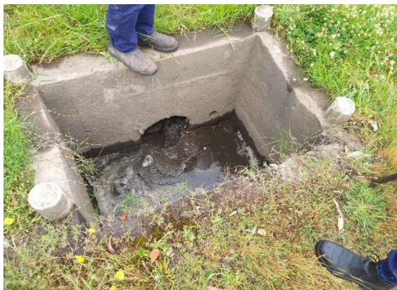
Figure 4 - Example of an absorption pit on Quay Road. Note the sediment build up in the base of the pit.
