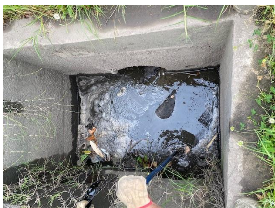
Figure 6 - Example of an absorption pit on Quay Road. Note the sediment build up in the base of the pit.
