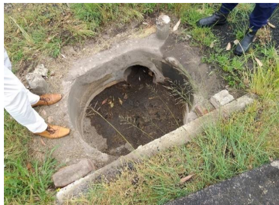
Figure 5 - Example of a stormwater pit on Quay Road with a concrete base.
