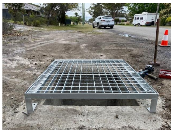
Figure 7 - New absorption pit installed outside 2 Quay Road to improve localised drainage.
