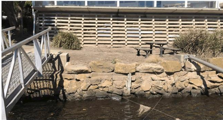
Figure 30. The original sea wall which is different to the rest of the sea wall. There is evidence of early construction such as the remains of a post seen in this picture.
