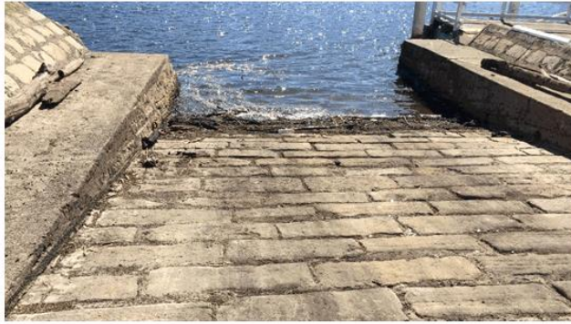
Figure 32. Sandstone slipway and retaining walls.
