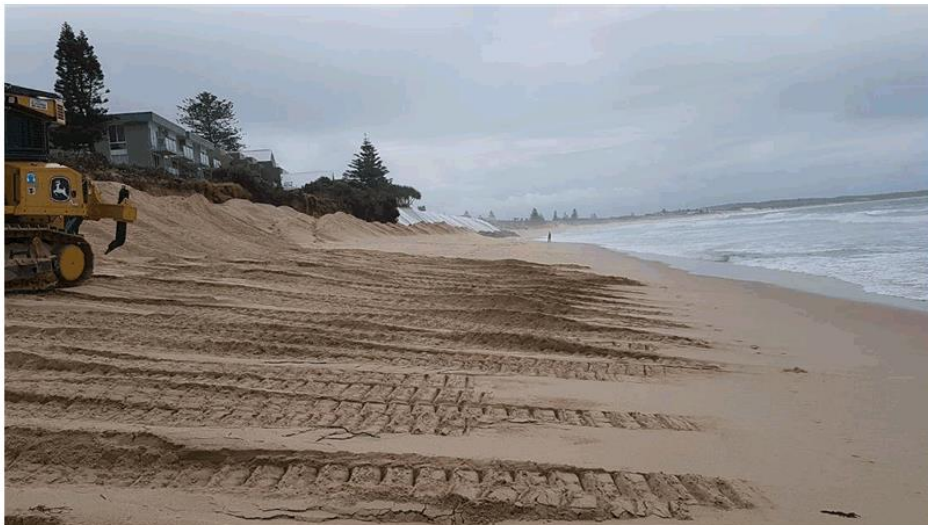
Figure 4-10: View of the beach nourishment site and shaping of the nourishment sand by dozer. The beach nourishment site comprised both an estuary beach and an open coast beach
