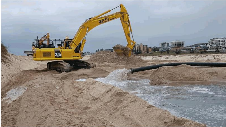
Figure 4-9: View at the settling pond showing discharge of the slurry and management of the dredged material into a stockpile by excavator. The dewatered material was then loaded into trucks for transport to the nourishment site.
