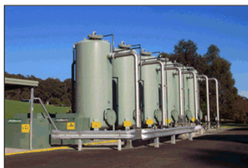
Tertiary Filters Callala WwTP
