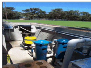
Pumping & disinfection system Huskisson Soccer Field
