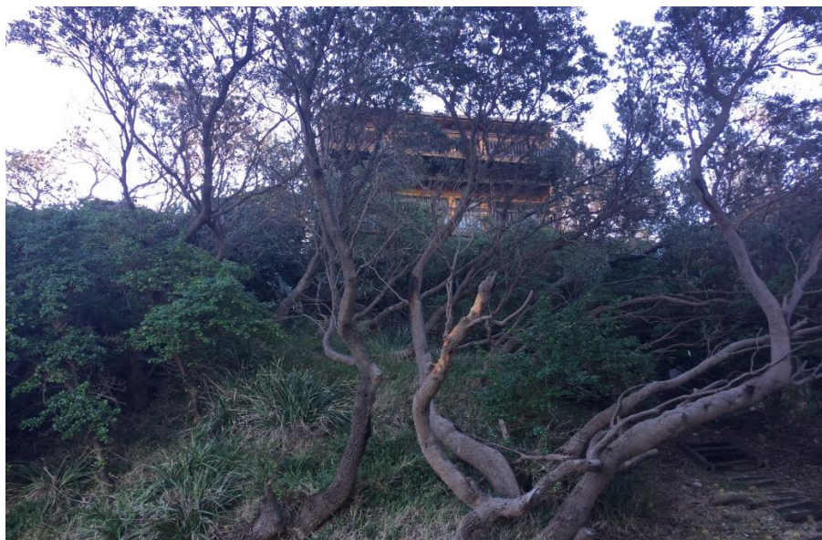
Figure 6 – Photos of existing building from front and rear
