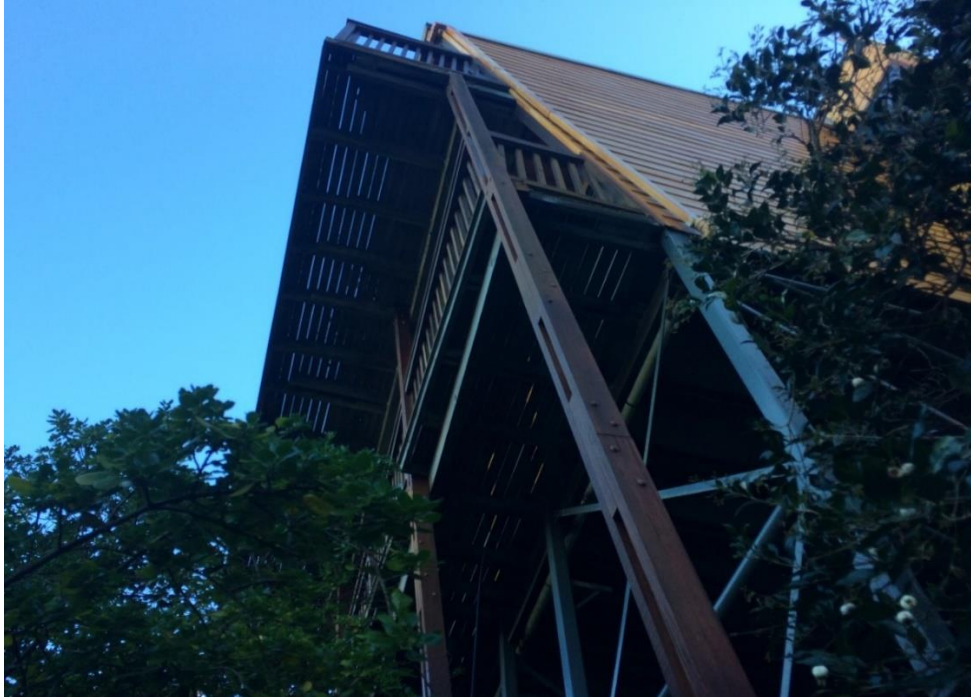
Figure 3 - Photos of existing structural elements
