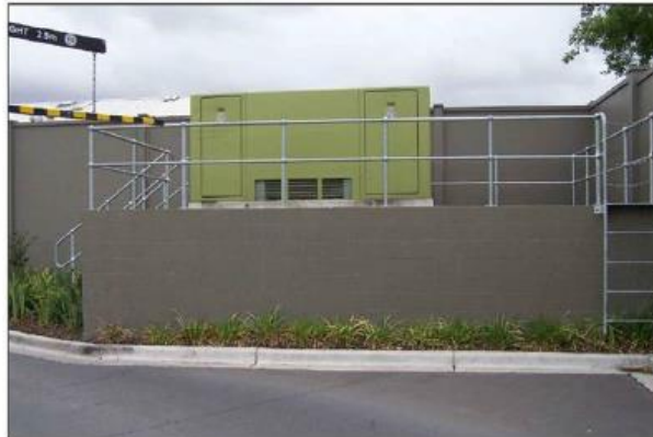
Figure 51 - Example substation raised above 1:100 flood level
