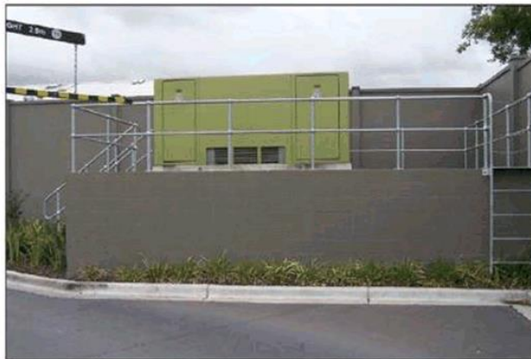
Figure 51 - Example substation raised above 1:100 flood level
