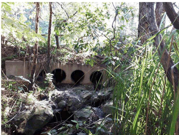
Picture 26- 375 RCP - Asset ID352470 + 375mm RCP Asset ID352471 + 3 Cell road culvert
