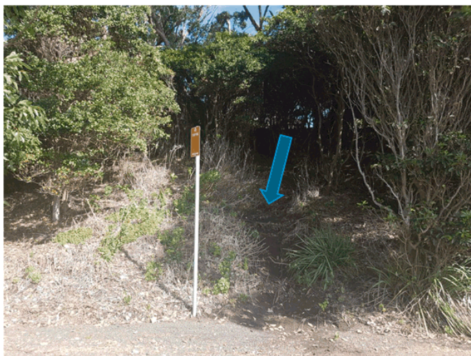
Figure 2-11 – Embankment behind road to west of boat ramp. Note area devoid of vegetation where rainwater flows appear to have concentrated from the top of the embankment on 17 March 2017, flowing directly over the road and onto the beach (20 March 2017)
