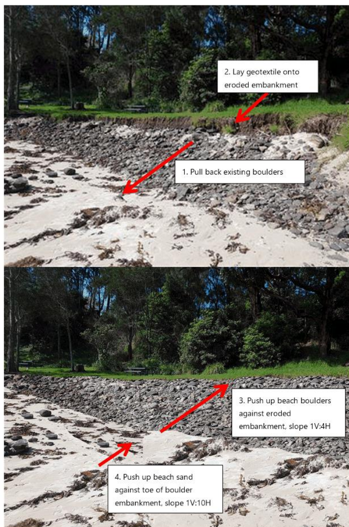
Figure 5-4 - East of Boat ramp, Top – existing; bottom – proposed (photo digitally altered). Proposed steps for remediation numbered on figure.
