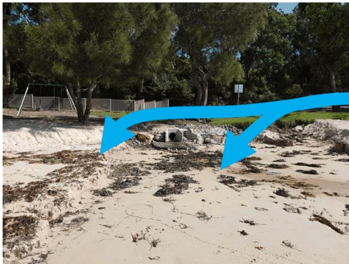
Figure 2-6 – Scour and beach erosion at playground area caused by overland stormwater flows from the road
