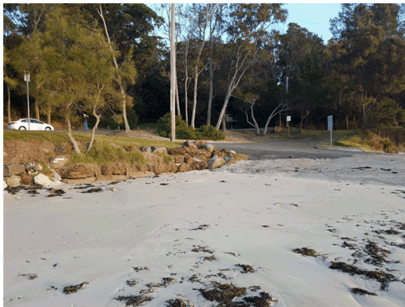
Figure 10 – Existing rock protection immediately east of main boat ramp, measured on site to have a median diameter of 800 mm (17 May 2018).
