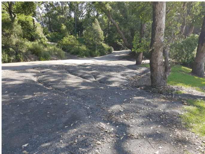
Figure 2-12 – Overland flow onto beach and playground area from steep approach roadway from the west, causing erosion on the beach near the existing playground area
