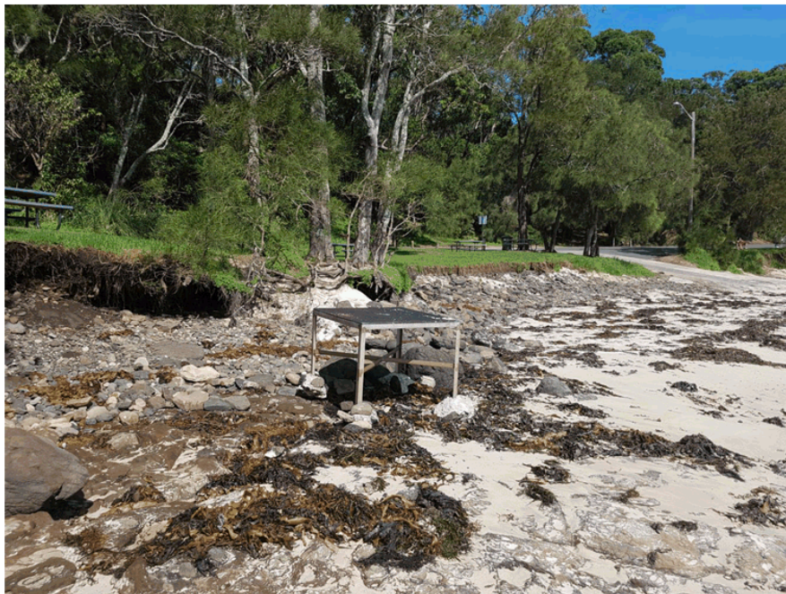
Figure 2-3 – Erosion at eastern end of Bendalong Boat Harbour Beach. Note fish cleaning table, exposed rock boulders and underlying bedrock, and boat ramp at background
