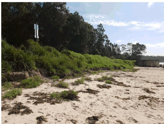
Figure 2-7 – Western end of Boat Harbour Beach. Note undermining of embankment toe by wave action and back beach area overgrown with exotic weeds (20 March 2017)
