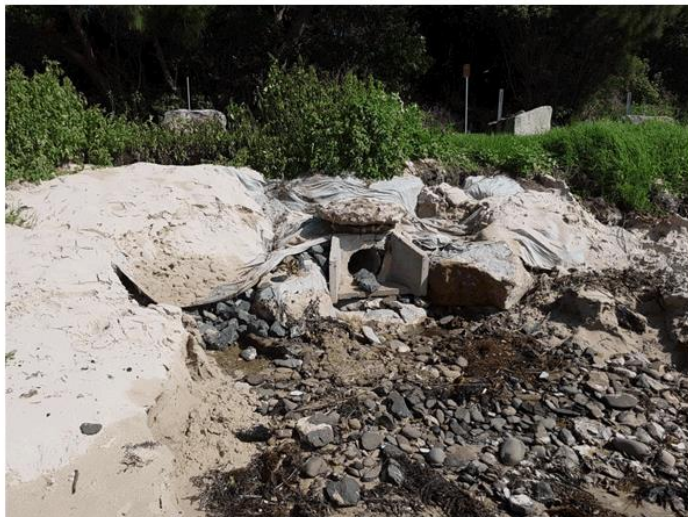
Figure 2-4 – Stormwater outlet to west of boat ramp – note poor condition, exposure of geotextile and concrete reinforcement and scour on the beach berm
