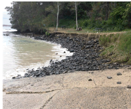
Photo 6: Location of shoreline protection works at eastern end
