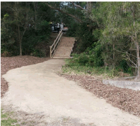
Photo 1: Stage 1 beach access steps at the western end of the beach
