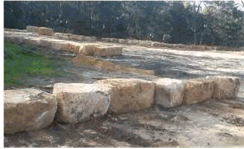
Photo 3: Concept for midden protection barrier with some form of fencing bolted to the top of the rock. Interpretive information about the Aboriginal cultural heritage will be incorporated into the barrier.
