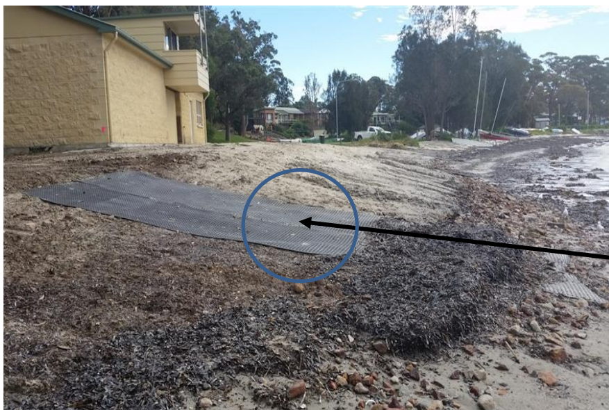
Photo 2: Completion photo showing finished level and holey belt access ramp
