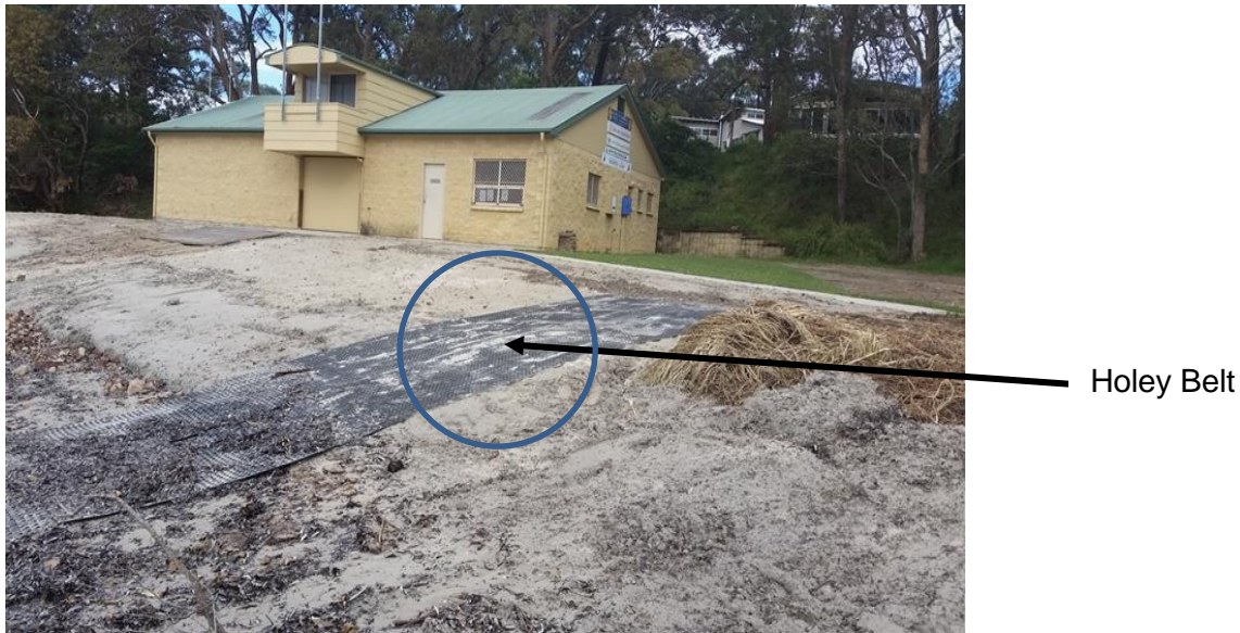
Photo 3: Completion photo showing finished level and trial holey belt access ramp
